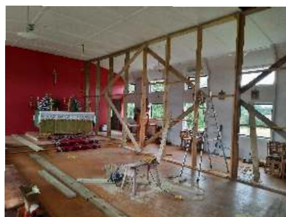
Progress at the Catholic Church
